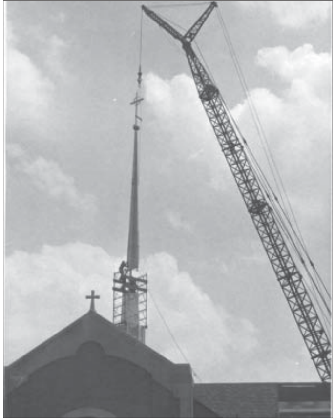
A boom crane positions the steeple
