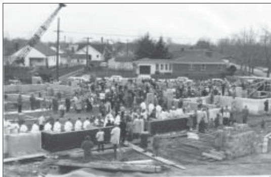
The laying of the cornerstone
