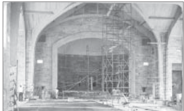
Church's structure takes shape
